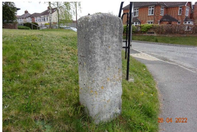
The St Francis milestone: the benchmark can be seen on the left side
